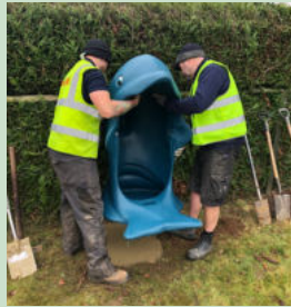
Installing new bins
