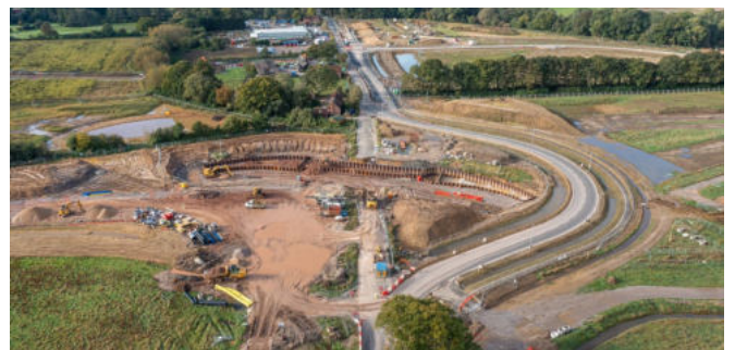
Woodhouse Lane looking south - Temporary link Road and underpass excavation
