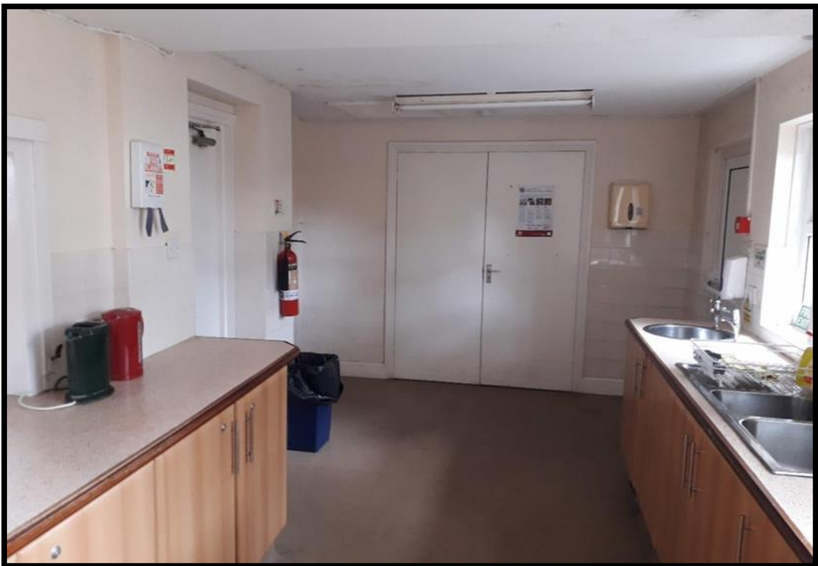
Kitchen viewing south towards the stud wall (to be removed).
